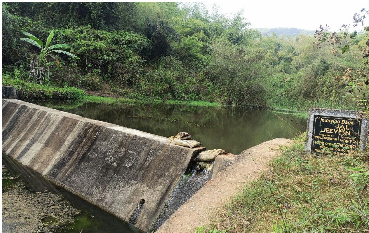
Figure 10: Check dam constructed in the Nakamudia village
