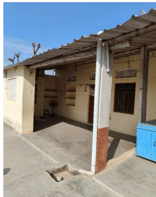
Figure 5: RRWHS constructed at home of beneficiaries in Devariya
