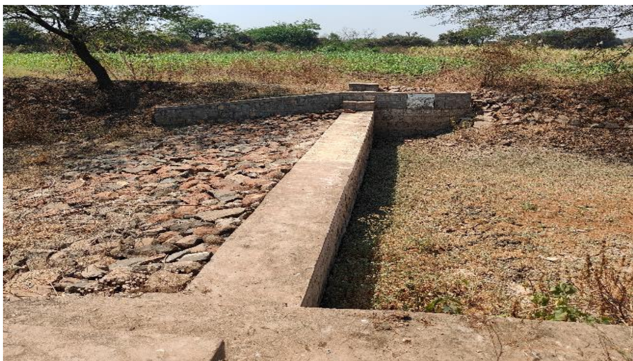
Figure 7: Check dam constructed by the project in Pattan village
